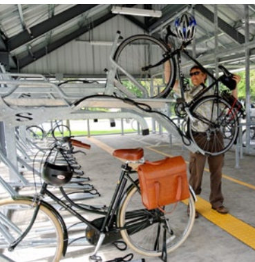
Figure F-18: Double-Decker Racks
