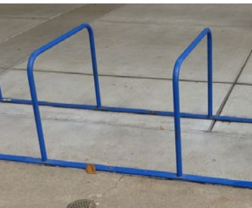
Figure F-10: Racks Mounted on Rails
