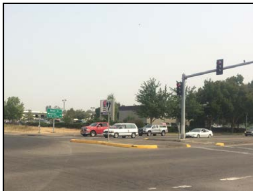
Figure 52: Pedestrian medians reduce unprotected crossing distances.
