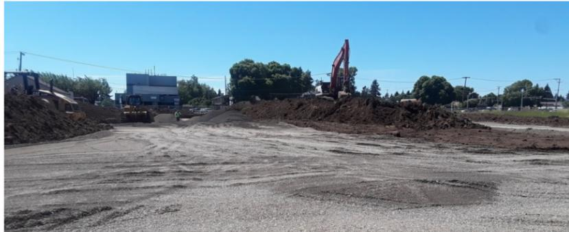
Pictured Above: Aggregate base being laid for the new transit station on May 28, 2020
