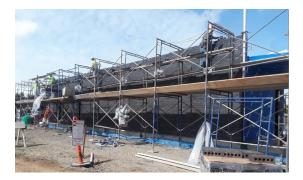
During the latter part of September, the masons were on site and completed the brick exterior walls of the driver relief building.
